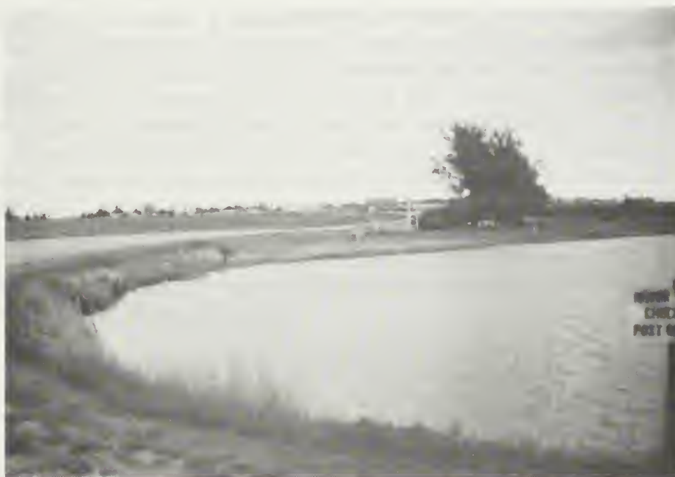
Figure 9 - North view of Raymond Reservoir
